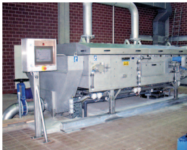
Thickener installation for up to 100 m 3 /h
