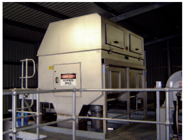
ROTAMAT® Rotary Drum Screen RoMesh® for optimal separation of very fine particles
