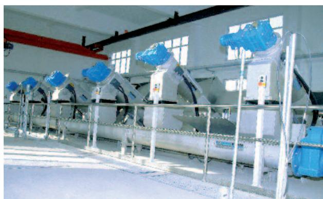
*ROTAMAT® Membrane Screen RoMem: screening in the inlet to membrane wastewater treatment plants*
