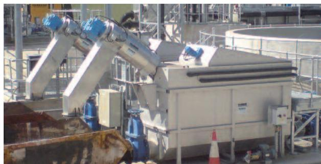
*ROTAMAT® Membrane Screen RoMem: tank installation*
