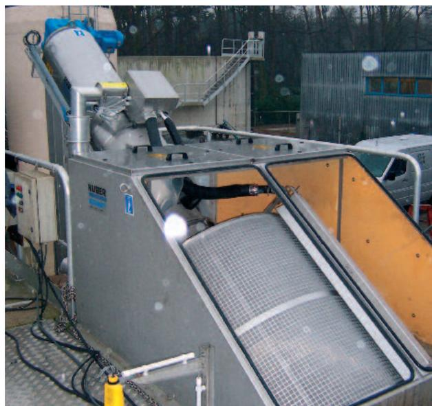
*Outdoor installation for removal of hairs and fibres prior to a hollow fibre membrane plant*
