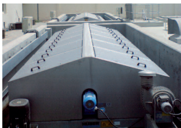
RoDisc® Rotary Mesh Screen with 20 discs installed in a concrete tank
