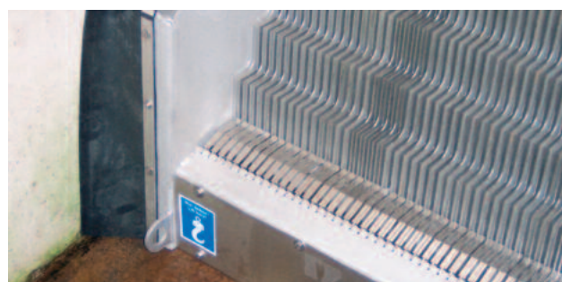
STEP SCREEN® Vertical SSV installed in a channel
