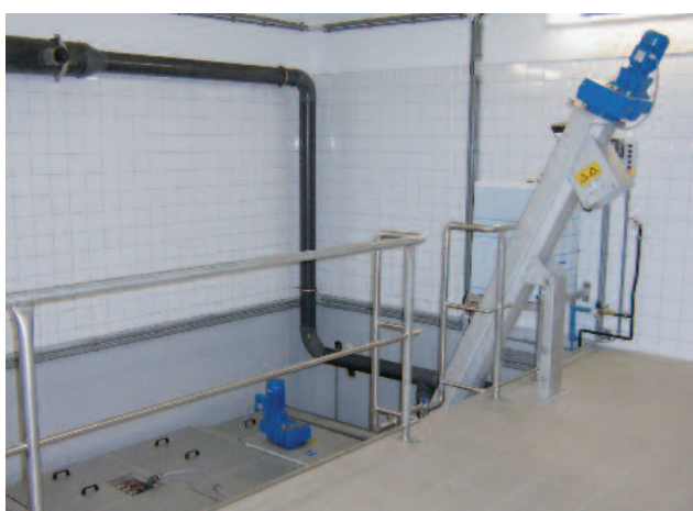
Integrated grit washing at the end of the ROTAMAT® Complete Plant Ro5
