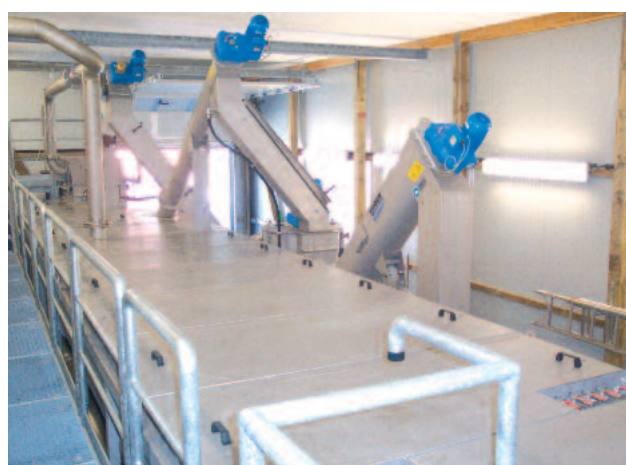
Odor-encased screenings discharge from the ROTAMAT® Complete Plant Ro5
