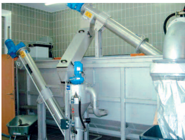
Classifying screw with subsequent HUBER Grit Washer RoSF 4/tC
