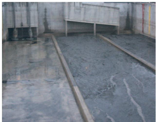
*Efficient removal of sediments with tipping buckets*
