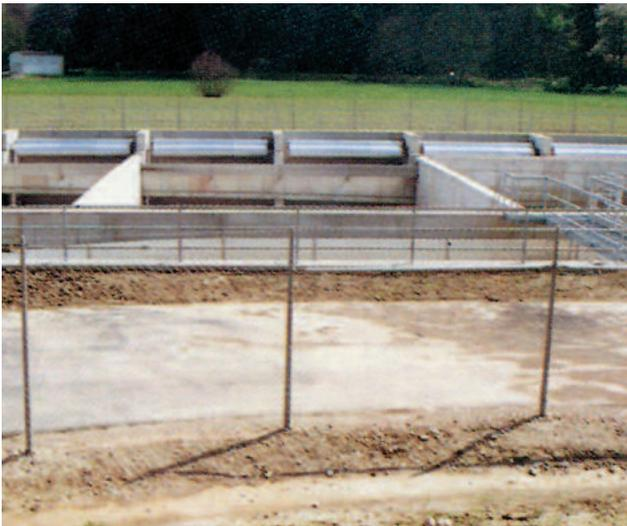
*Stormwater holding sewer with integrated chamber for installation of tipping buckets*
