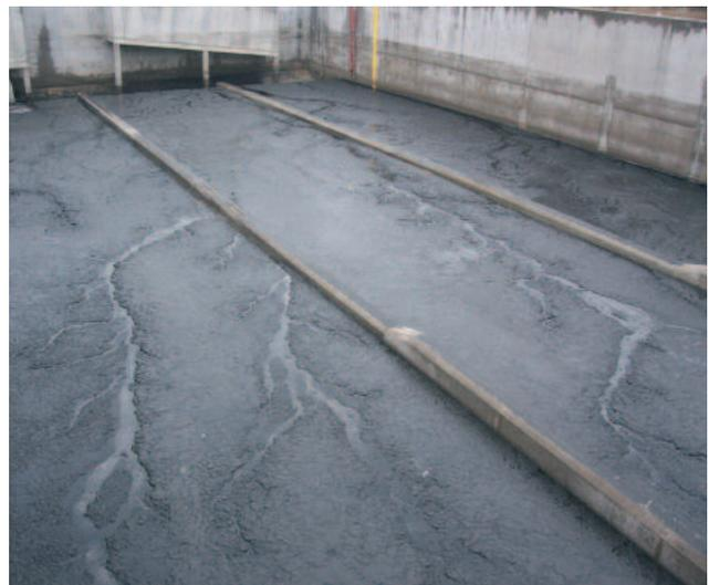
*Sediments in the stormwater tank after an impoundage event*
