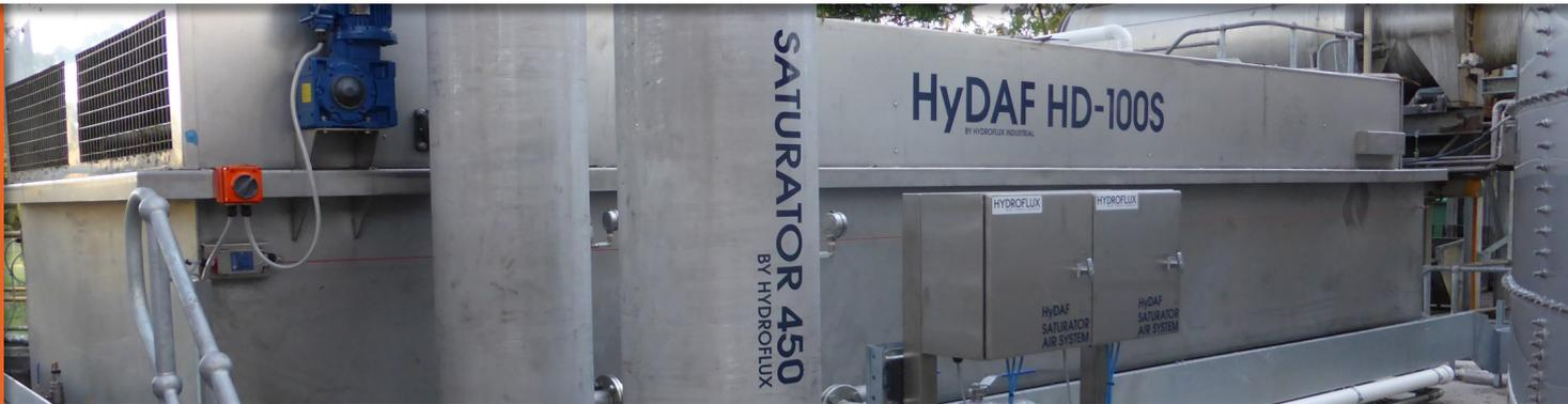
The Hydroflux HyDAF HD range of DAF systems offer superior performance in terms of wastewater quality and sludge dryness.
